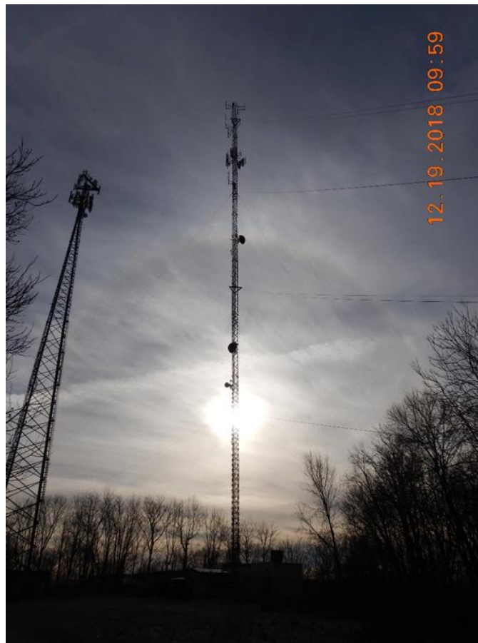
Figure 7: Photograph showing the telecommunication tower considered for stray current corrosion survey.
