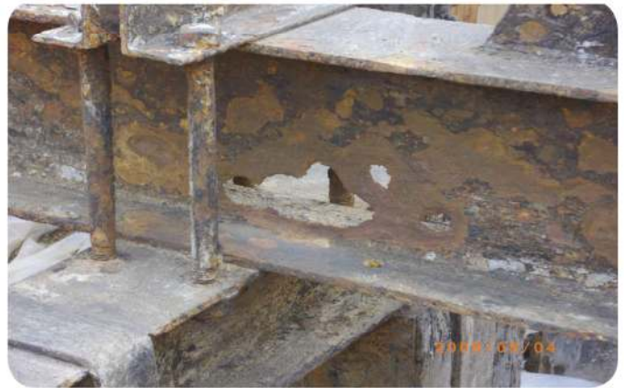
FIGURE 5 T&D towers on farmland are subjected to accelerated corrosion from corrosive ions.
