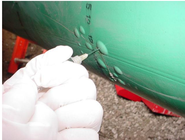
Figure 6: Blister liquid extraction - high pH solution due to cathodic delamination.
